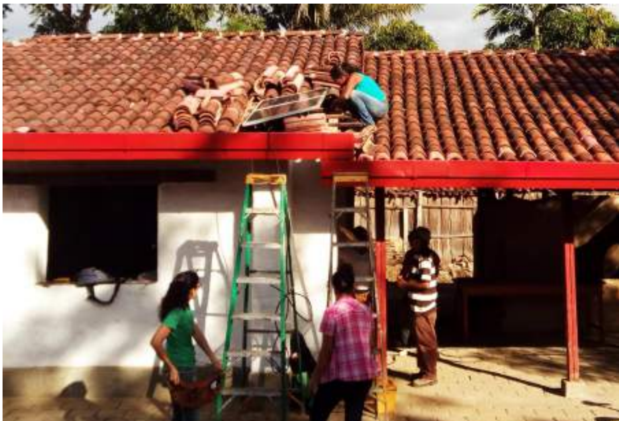
Fig.5/ Installation and maintenance of solar photovoltaic energy systems course, 2016, AMCC.
